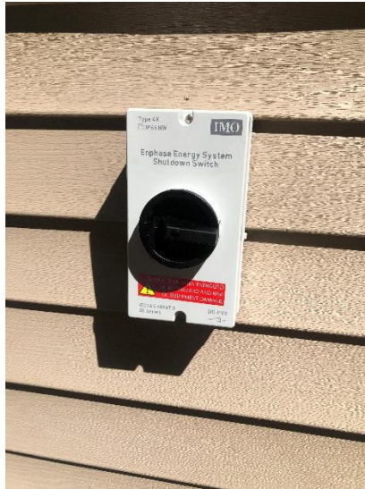
Figure 6: Emergency Disconnect Switch on back of garage
