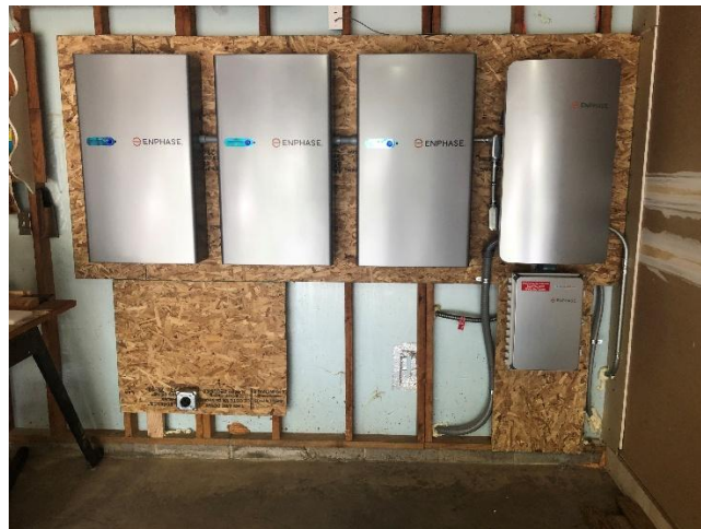
Figure 5: Solar Installation equipment inside garage
